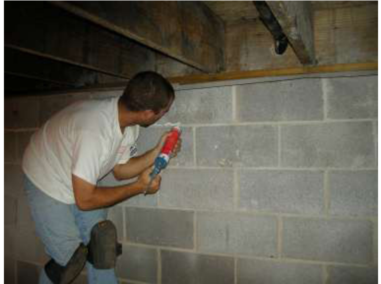
Applying the adhesive bead
