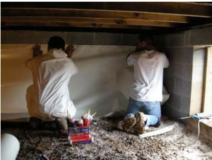
Applying the wall material
