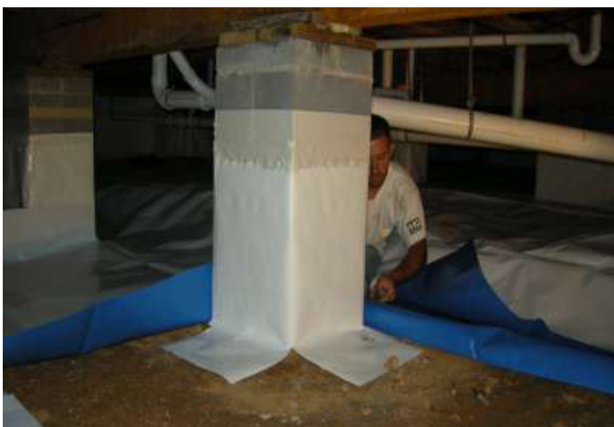
Installing the Floor Material Around a Pier.
